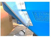
10 – Install the remaining bolts in the brackets and the top plate.
